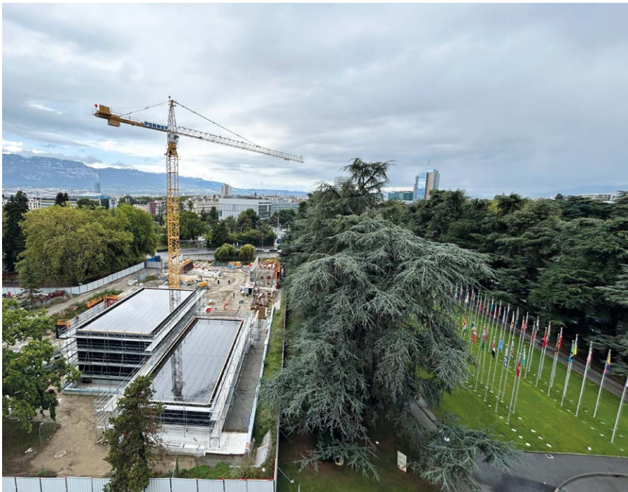
The construction of the Portail des Nations Visitor Centre at UN Geneva advances ahead of its planned opening in 2026. ©UN Photo: François Vioud
