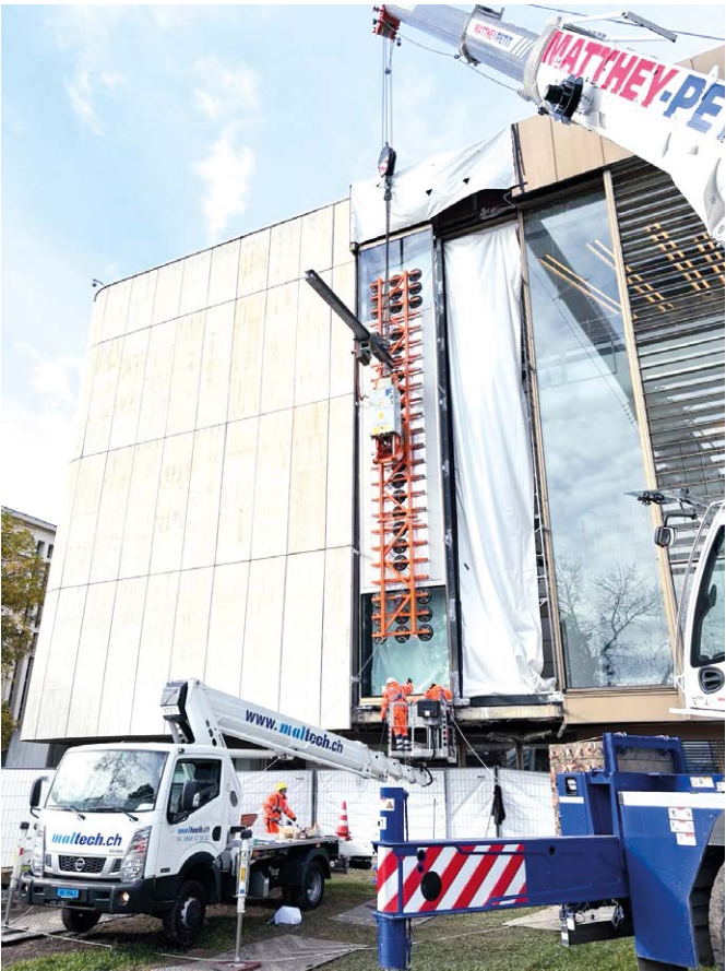
As part of the preparatory works of the Strategic Heritage Plan, two of the existing double-glazed windows are removed by a contractor. ©UN Photo: Strategic Heritage Plan
