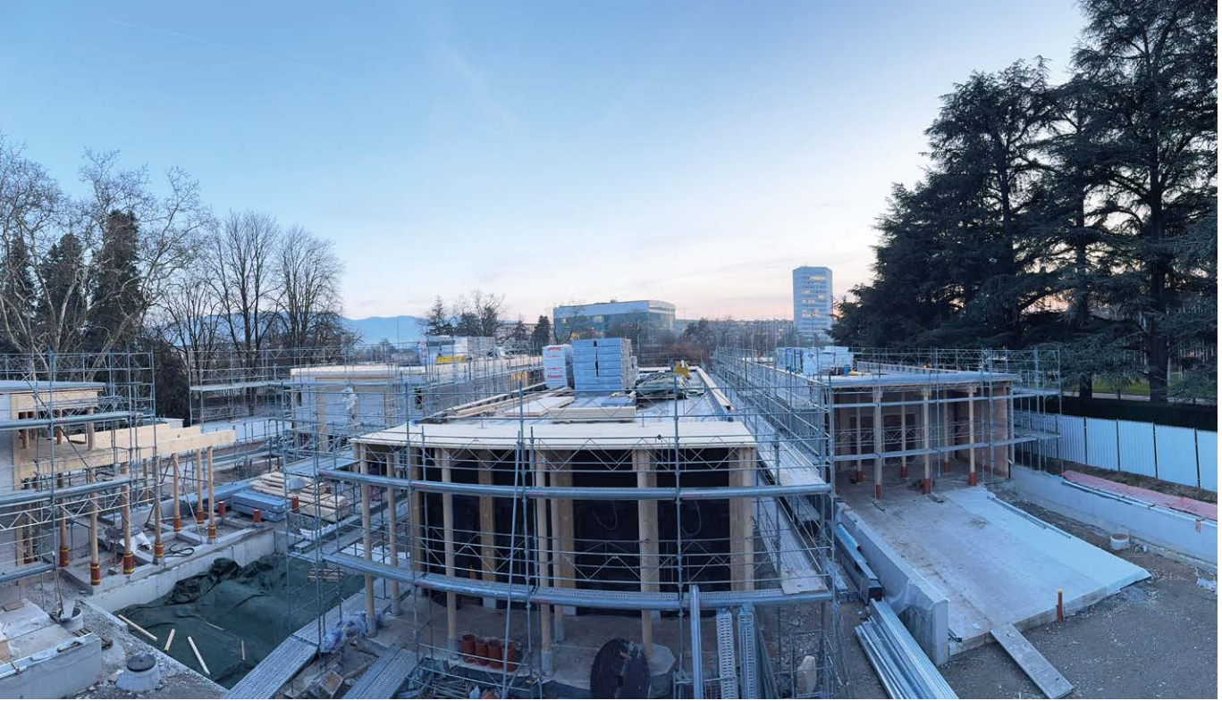
The Portail des Nations Visitor Centre, shown here under construction, is expected to open in 2026. ©UN Photo: Charbel Jabbour
