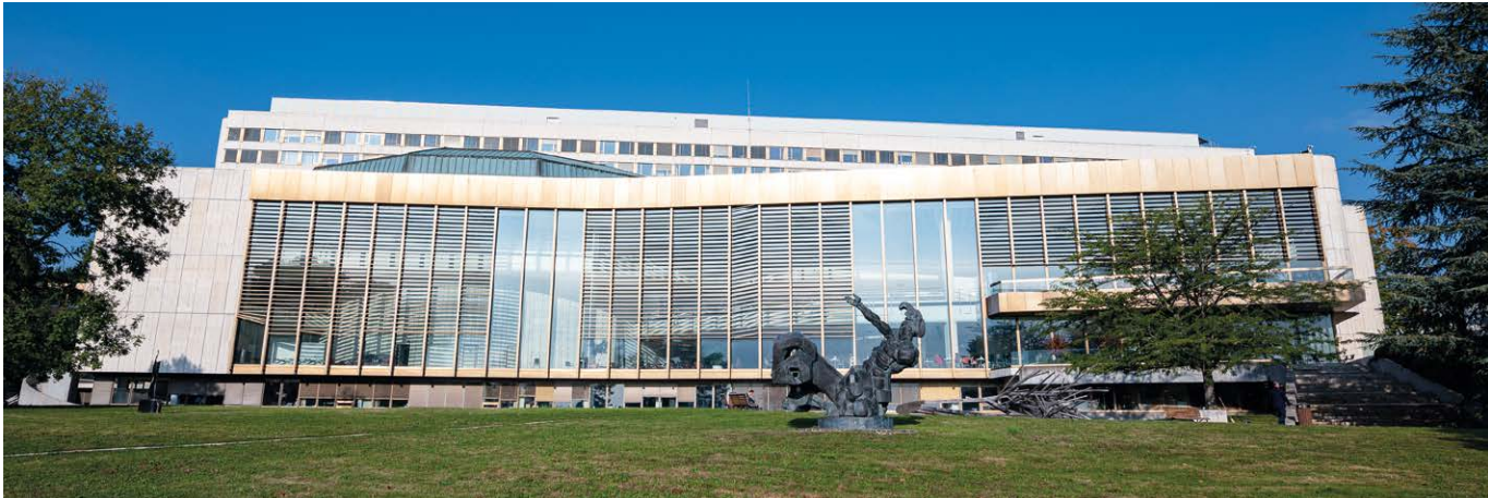
The lakeside façade of Building E dates from the early 1970s and includes 24 large, double-glazed windows. ©UN Photo: Matija Potocnik
