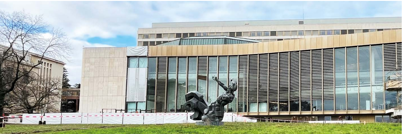
A mock-up of the renovated façade windows is installed. Building and heritage experts will review the mock-up before launching the production of the rest of the windows that will constitute the renovated façade. ©UN Photo: Strategic Heritage Plan
