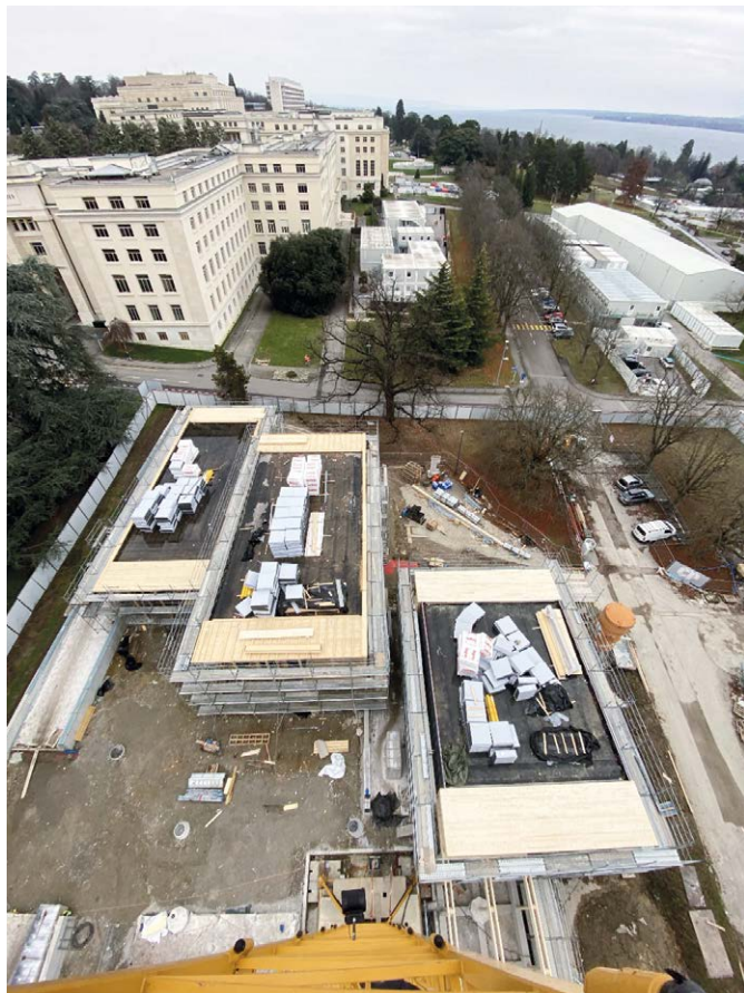
The construction site of the new Portail des Nations Visitor Centre, viewed from a crane. ©Charles Pictet Baptiste Broillet Architectes Associés
