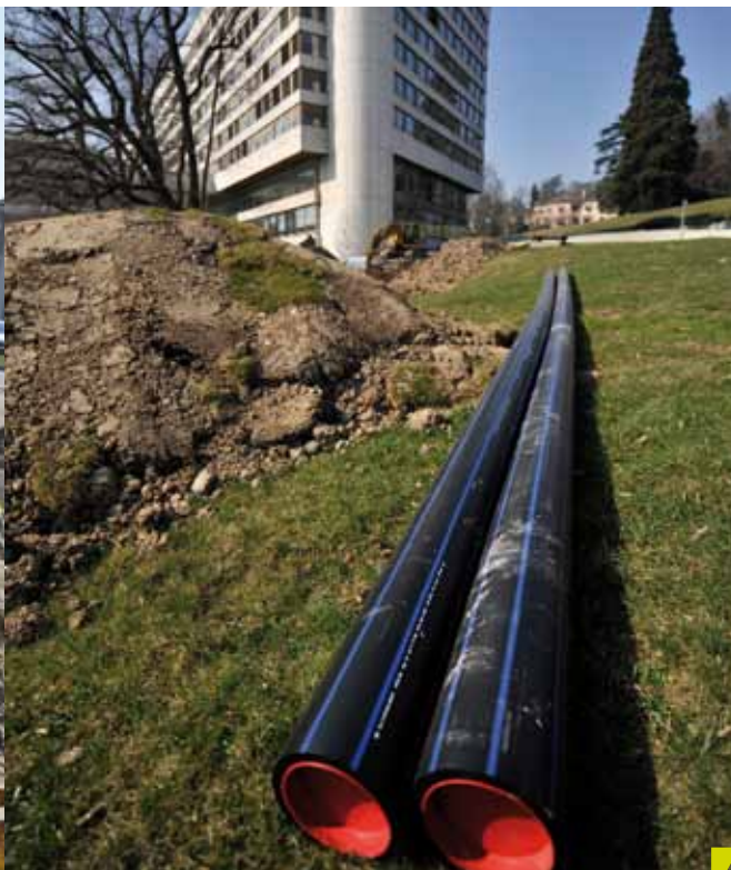
The Natural Gas Project construction site.
