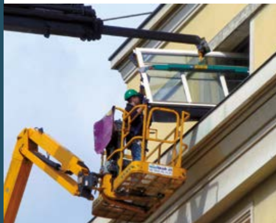
Window replacement at UNOG, 20 March 2013 (UN Photo/Central Support Services)
