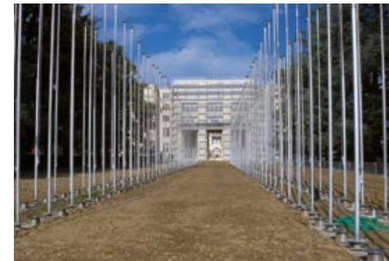
The Allée des Nations under renovation, 19 October 2013 (UN Photo/CSS)
