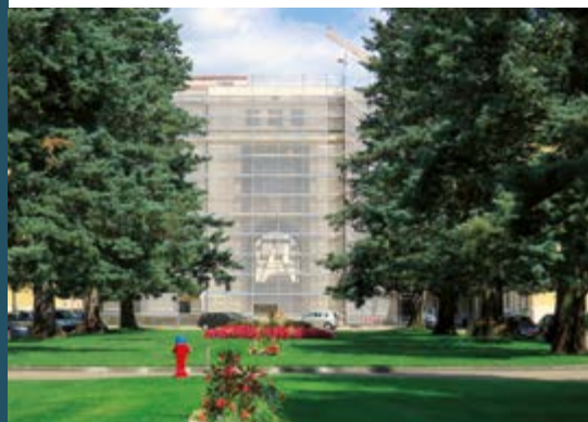
Building works to increase energy efficiency at UNOG, 10 August 2013 (UN Photo/ODG)
