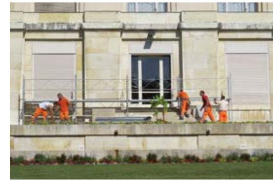
Window replacement at UNOG, 6 July 2013 (UN Photo/ODG)
